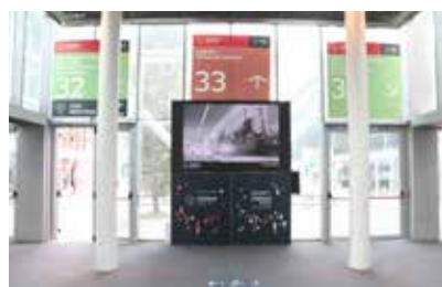
Services Centre glass wall facing halls 31/32
